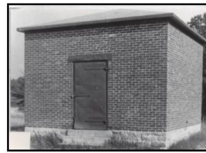
23. Magazine Storage, Behind the Old Stone Barracks
