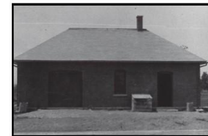
26. Ordinance Office and Storehouse, 29 Washington Road
