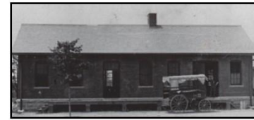
27. Carpenter and Blacksmith's Workshop, 31 Washington Road
