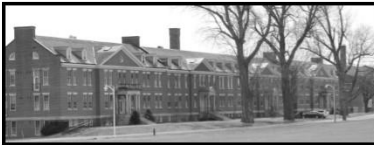
12. Enlisted Men's Barracks, 64-70 U.S. Oval
